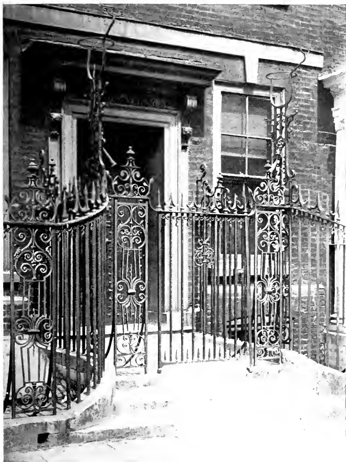
232. Wrought-Iron Gates, Great Ormond Street.
